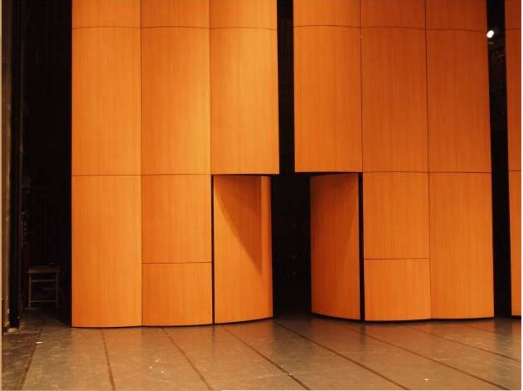
3.4 Double doors allow access of large equipment.
